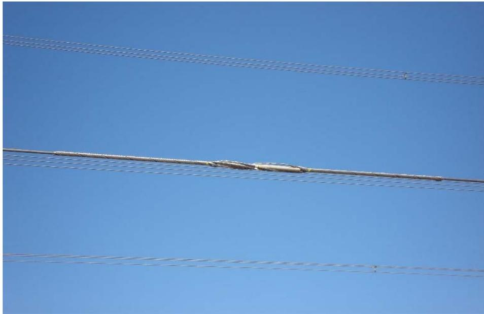
**Mid-span splice shunt.**
