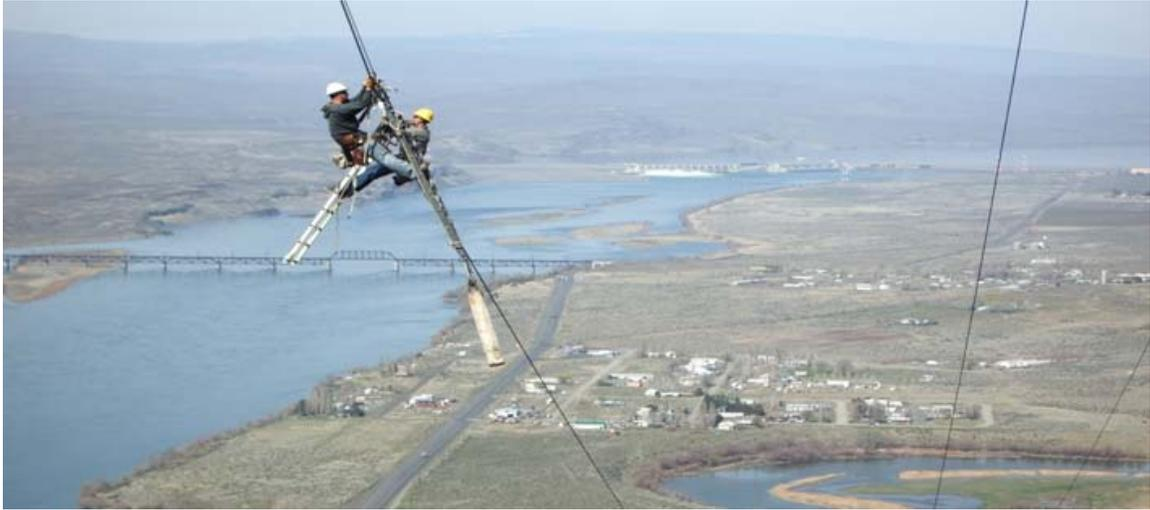
**BPA crews install a dead-end high-temperature shunt above the Columbia River.**
