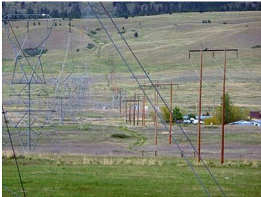
The proposed rebuild of the 115-kilovolt Kalispell-Kerr transmission line is part of BPA's commitment to maintain reliable electrical service and to reduce potential safety risks to the public and work crews. By rebuilding aging transmission lines when needed, BPA preserves the value of its transmission system, much of which is now nearing 70 years in age. If BPA chooses to proceed with the proposed project, construction would begin in the spring of 2016.
