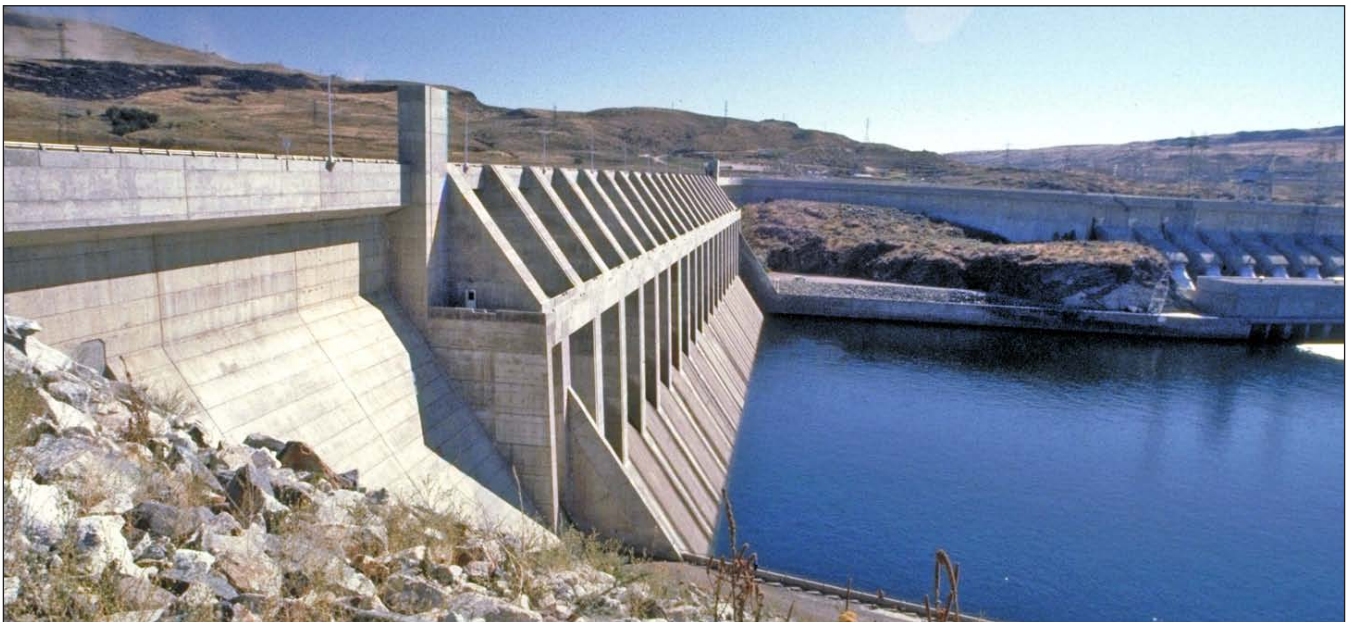
A state-of-the-art high performance fluorescent light system was installed at Chief Joseph Dam, saving 2 million kWh a year.
