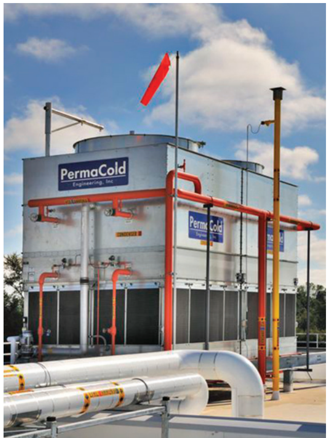
From seed to shelf, BPA's energy-efficiency programs target stages of the food production process. Top: An efficient irrigation system reduces water and energy use. Bottom: The smart refrigeration system at the SnoTemp Cold Storage facility can use more or less energy, as needed, to help balance power supply and demand.
