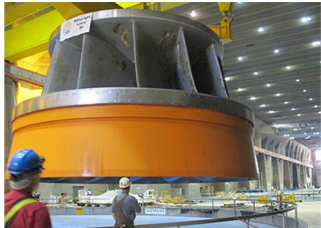
*BPA and the Bureau of Reclamation are overhauling the Third Power Plant at Grand Coulee Dam in northeast Washington. Here, workers remove a 3,000-ton hydroelectric turbine that had been producing power since the 1980s. All six turbines in the third powerhouse will be refurbished in the next 10 to 15 years as part of a \$275 million project funded by BPA ratepayers.*
