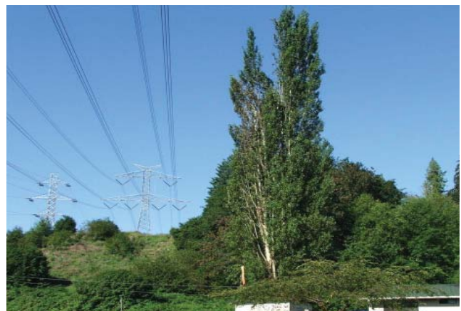
Electricity can "arc" to tall trees that are in close proximity to high-voltage lines and cause fires.
