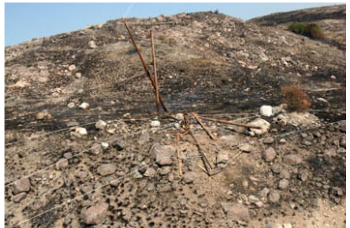
An Aug. 16 wildfire near Grand Coulee Dam damaged this wood pole structure on BPA's Keller Tap 115-kV line.
