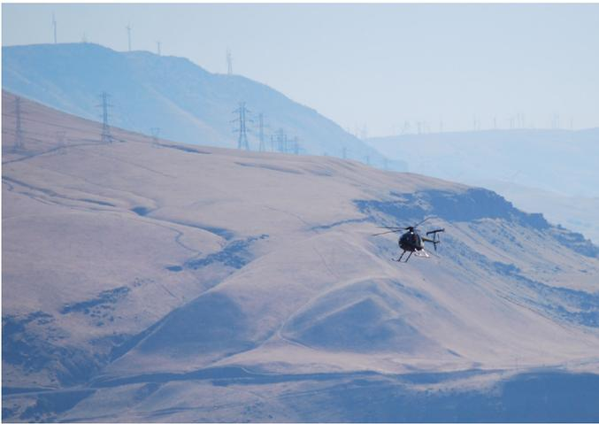
*A helicopter tows a rope across the Columbia River, near The Dalles, Ore., during construction of the new Big Eddy-Knight 500 kV line. The helicopter flew rope across the river to start stringing at the line's river crossing.*
